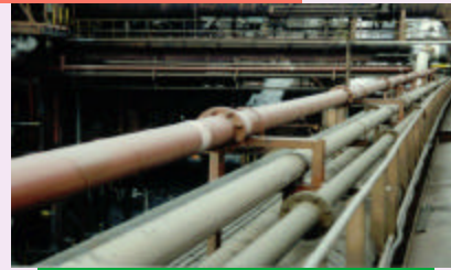
FLYASH PIPEWORK
